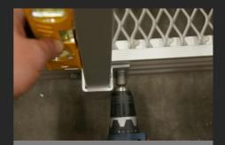
14. Place and level the rail. Tighten the screws for the railholder, always tighten the left screw first.
