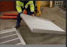
Lay down the next ramp section. Repeat 4-5 until desired length
