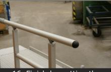
16. Finish by putting the plastic cap on the end part of the handrail.
